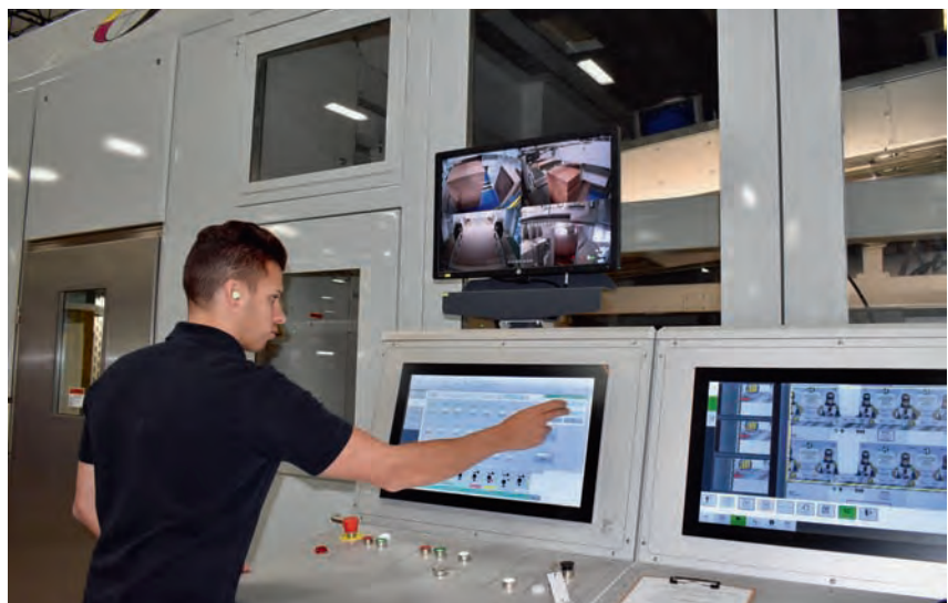
Operators monitor the Göpfert press from a central control station.
