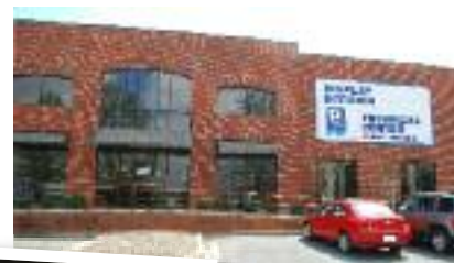
THE CONYERS, GA., FACILITY.
